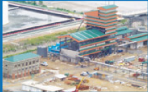
Kuching Health Inspector Institute Batu 7, Kuching, Sarawak (Inai Kiara Sdn Bhd)
